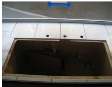
Figure 11 Fixture and sink cutouts
