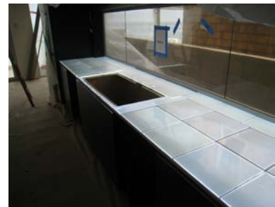
Figure 12 Installed counter SLABlite panels
