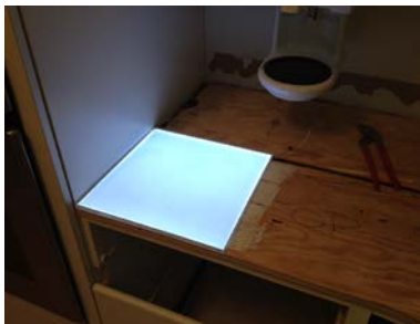
Figure 10 SLABlite tested, glued in place
