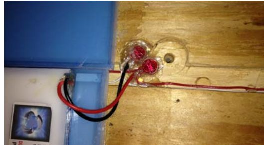
Figure 9 Connector / wires secured with hot glue
